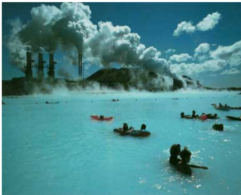
Iceland's Famous Blue Lagoon, Geo Power Plant & Production Fluid
